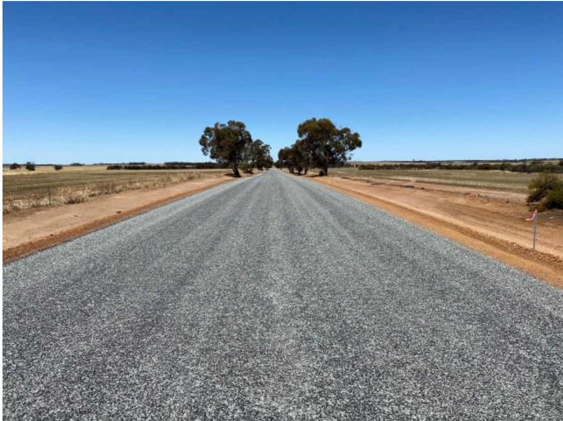
Final sealing of Yerecoin SE Rd for 2km after Reconstruction in early November 2020
