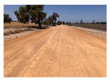
Old Telegraph Rd is approaching the completion of the Roads to Recovery program of vegetation and re-sheeting works for the 2km north of Bolgart West Rd. Shire staff have completed this work utilising local gravel and have stored the excess soil from the verge for rehabilitation on older gravel pit sites. White delineator posts are yet to be installed.
