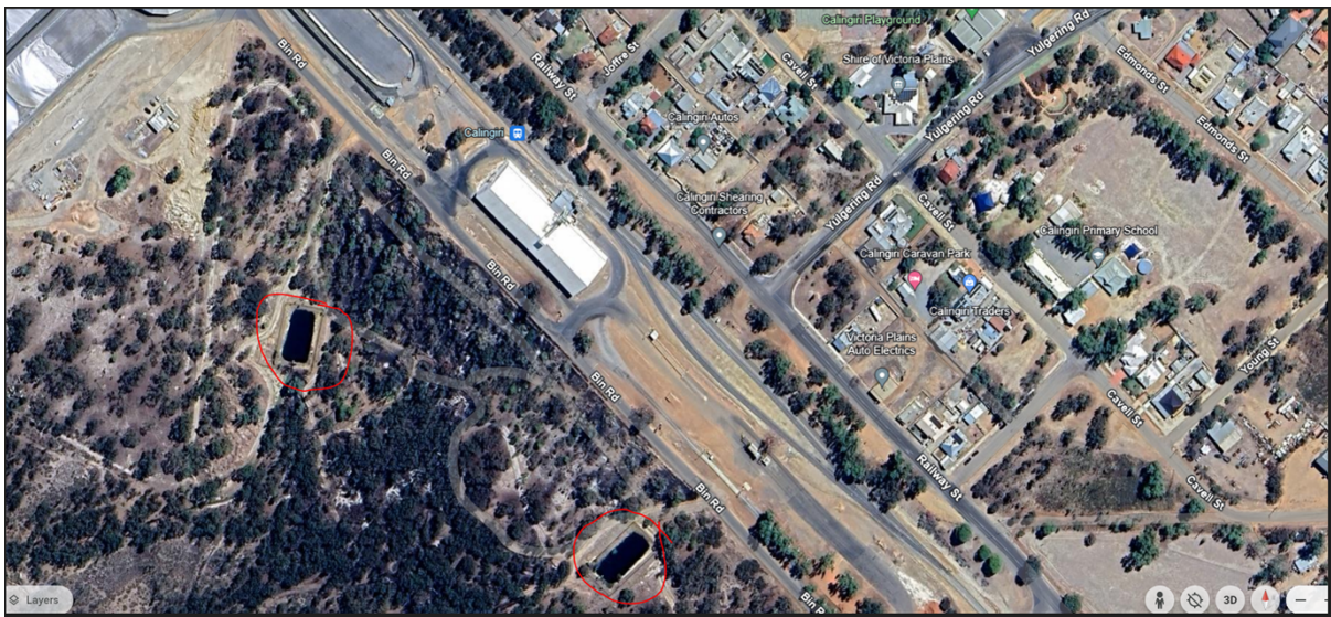
Figure 8: Calingiri sewerage ponds
