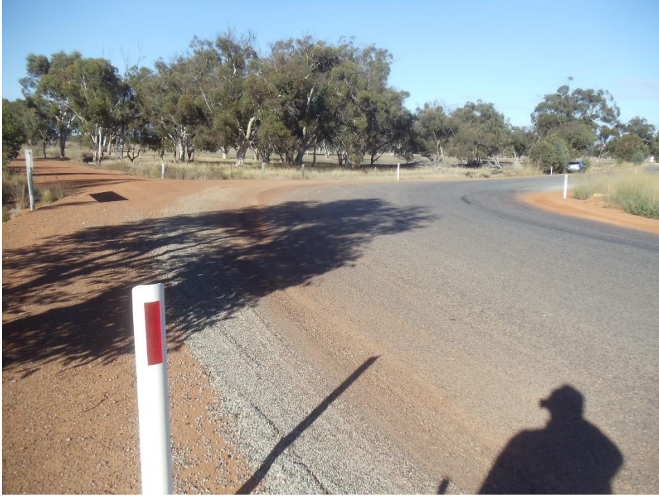
Note how tight bend
