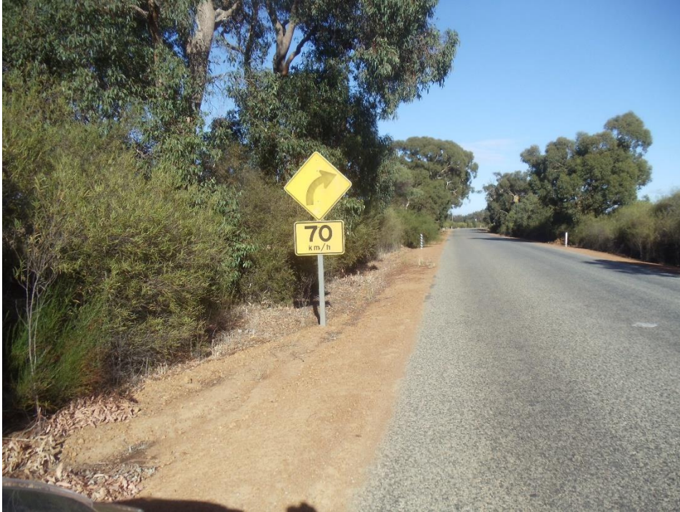
Looking west at start of right hand curve – note narrow gravel shoulder
