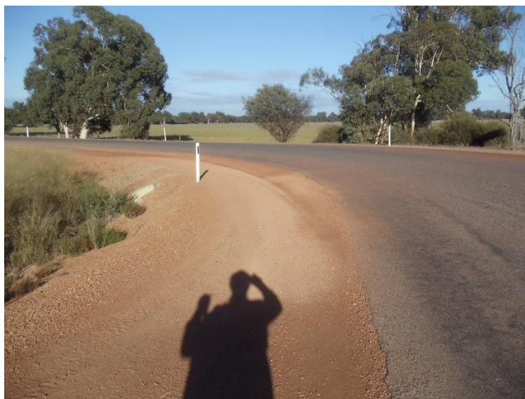
Note trucks running off road on inside of curve
