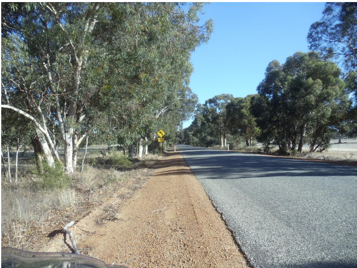
Looking west at start of left hand curve – note narrow gravel shoulder
