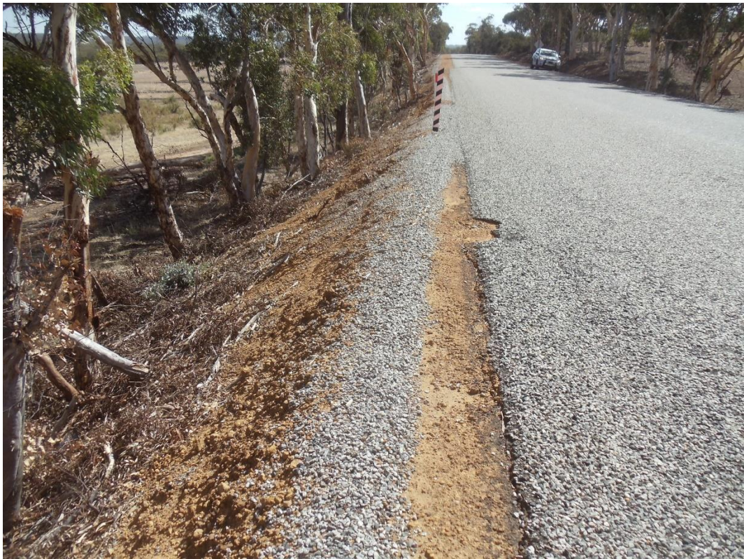
Looking east from southern side of the road - note narrow shoulder and steep batter. Note batter erosion
