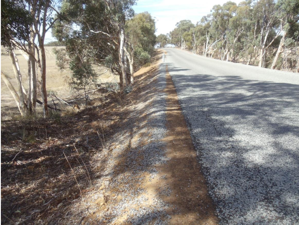
Looking east from northern side of the road - note narrow shoulder and steep batter
