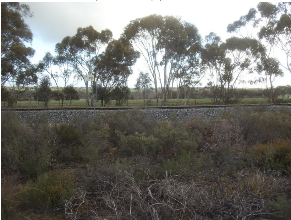
Proposed New alignment – looking west down – for Calingiri New Norcia just near Toodyay Bindi Bindi Road – 180 degrees around from above
