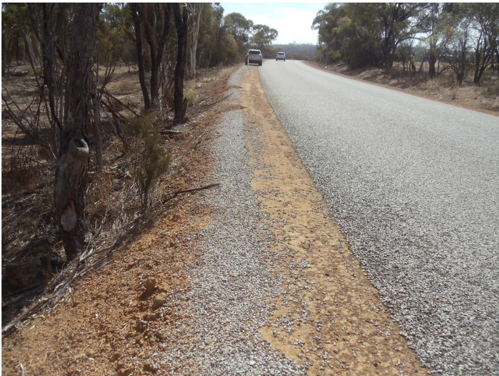
Looking west note narrow shoulder around curve
