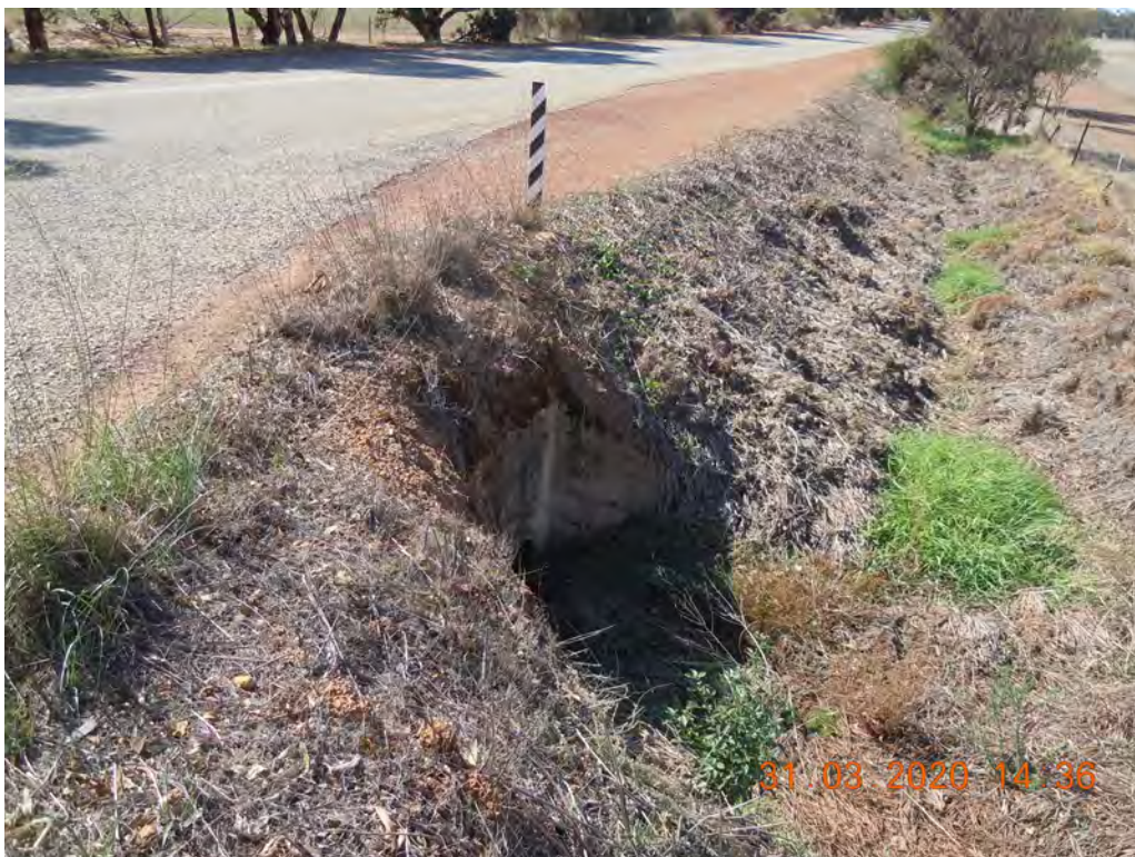
PHOTOGRAPH 30 - 6.17 SLK Mogumber Road culvert RHS 2 x 300RCP
