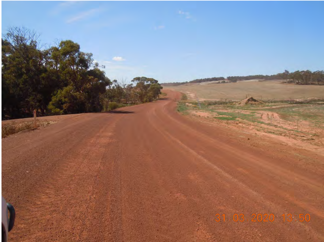
PHOTOGRAPH 11 2.56 SLK Cocking Road Looking north – note steep batters
