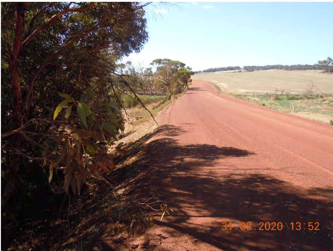
PHOTOGRAPH 12 2.53 SLK Cocking Road Looking north – note steep batters.
