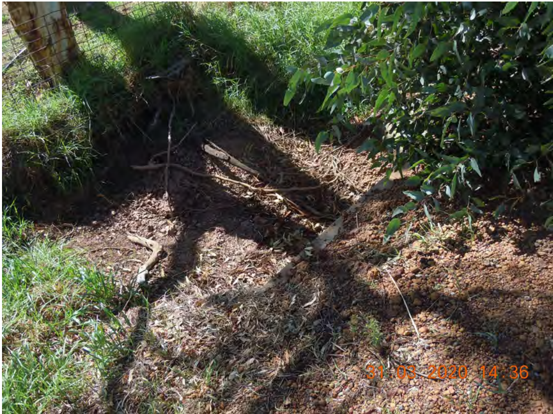
PHOTOGRAPH 32 - 6.17 SLK Mogumber Road culvert LHS 2 x 300RCP
