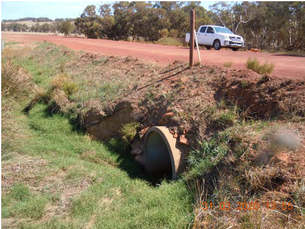
PHOTOGRAPH 14 2.44 SLK Cocking Road LHS 900 RCP 8.6m running surface
