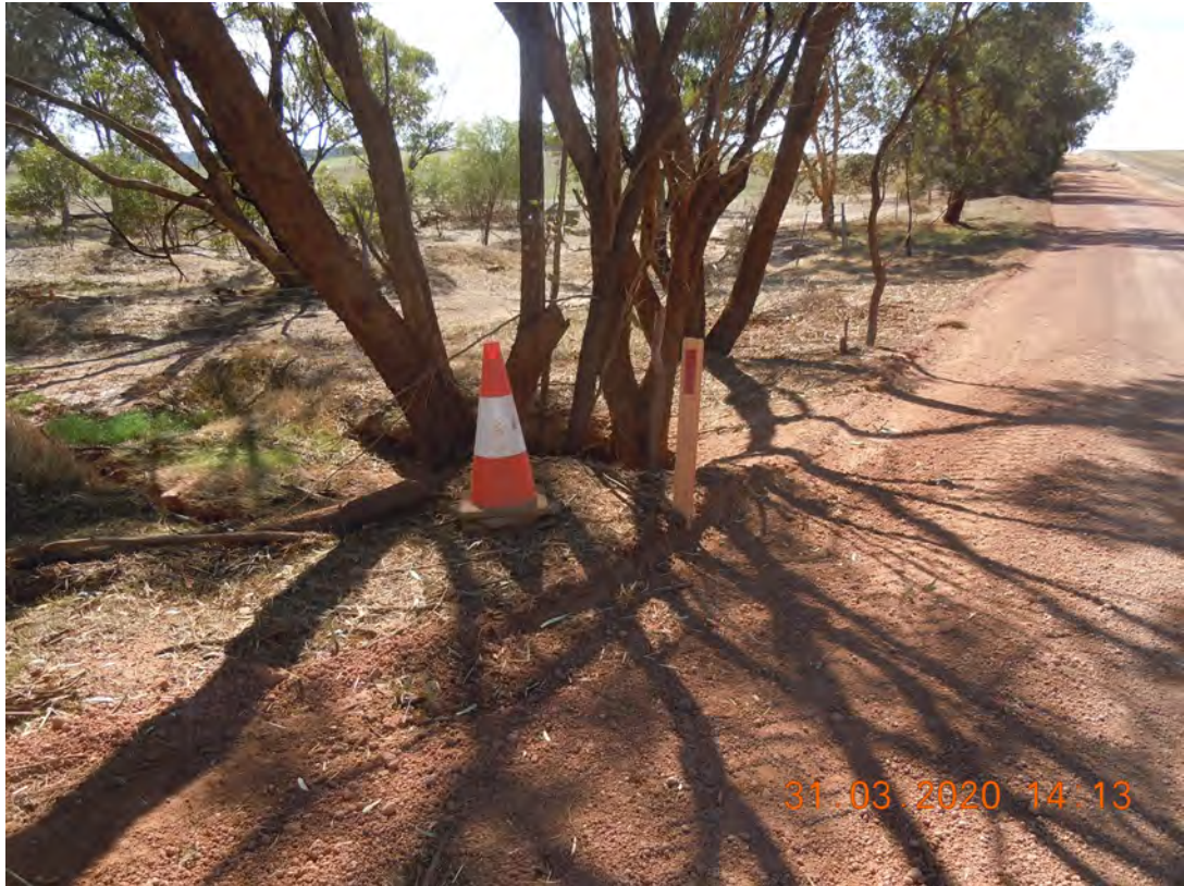
PHOTOGRAPH 23 - 1.22 SLK Cocking Road looking south culvert
