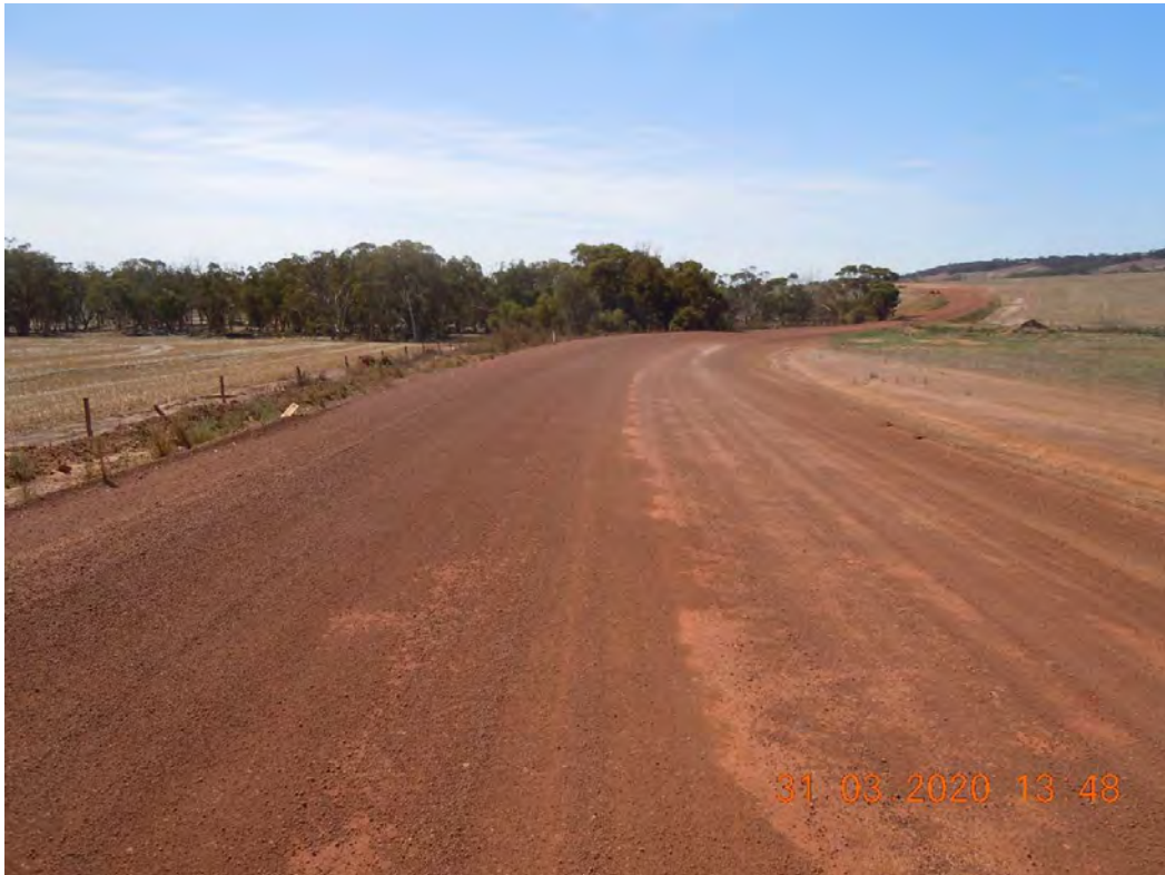
PHOTOGRAPH 1 SLK 2.66 Cocking Road looking north -Typical View
