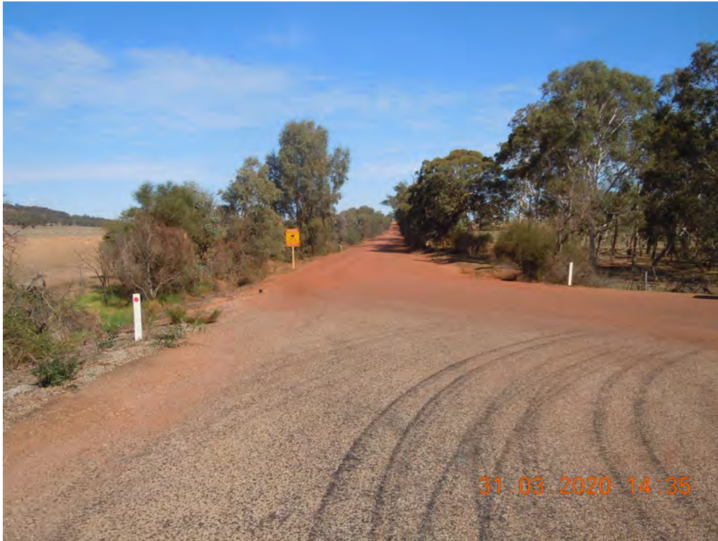
PHOTOGRAPH 29 - 6.15 SLK Mogumber Yarawindah Road looking south from Cocking Road Intersection down Cocking Road
