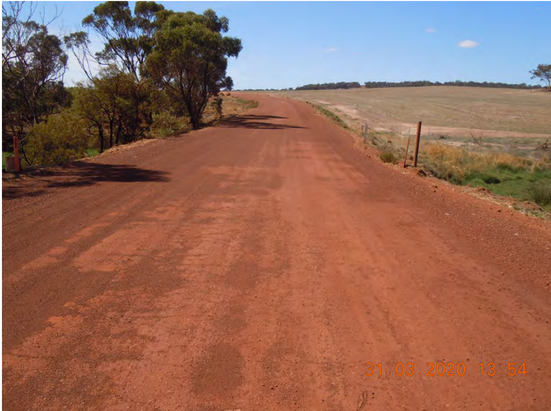
PHOTOGRAPH 13 2.44 SLK Cocking Road Looking north – culvert site – note steep batters.
