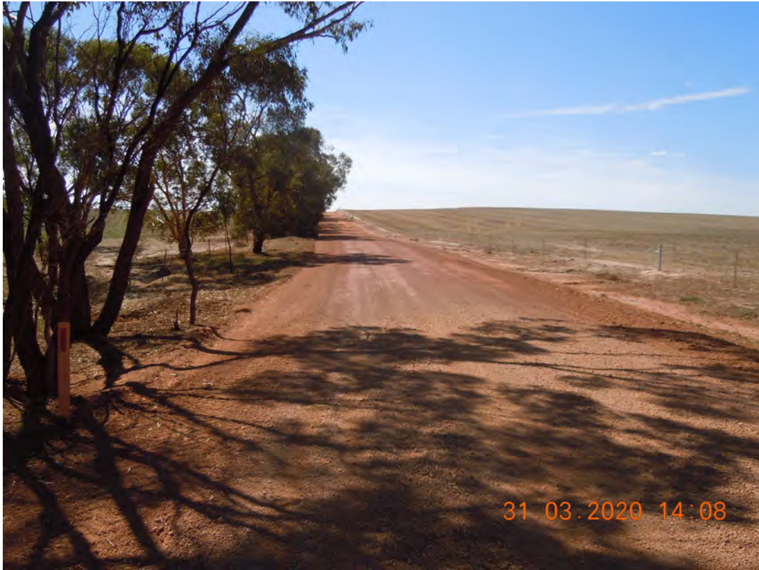
PHOTOGRAPH 19 - 1.22 SLK Cocking Road looking north from culvert
