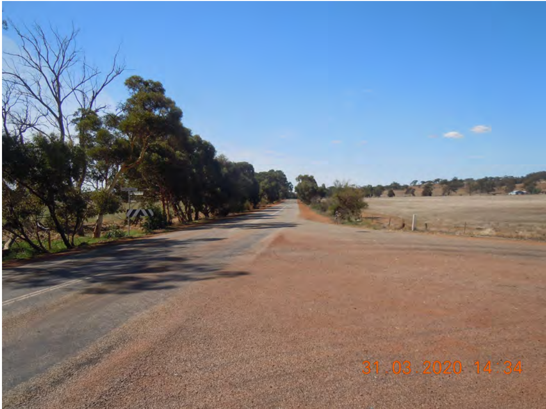
PHOTOGRAPH 25 - Mogumber Yarawindah and Cocking Road intersection looking east
