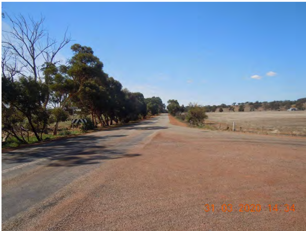
PHOTOGRAPH 3 - Mogumber Yarawindah and Cocking Road intersection looking east
