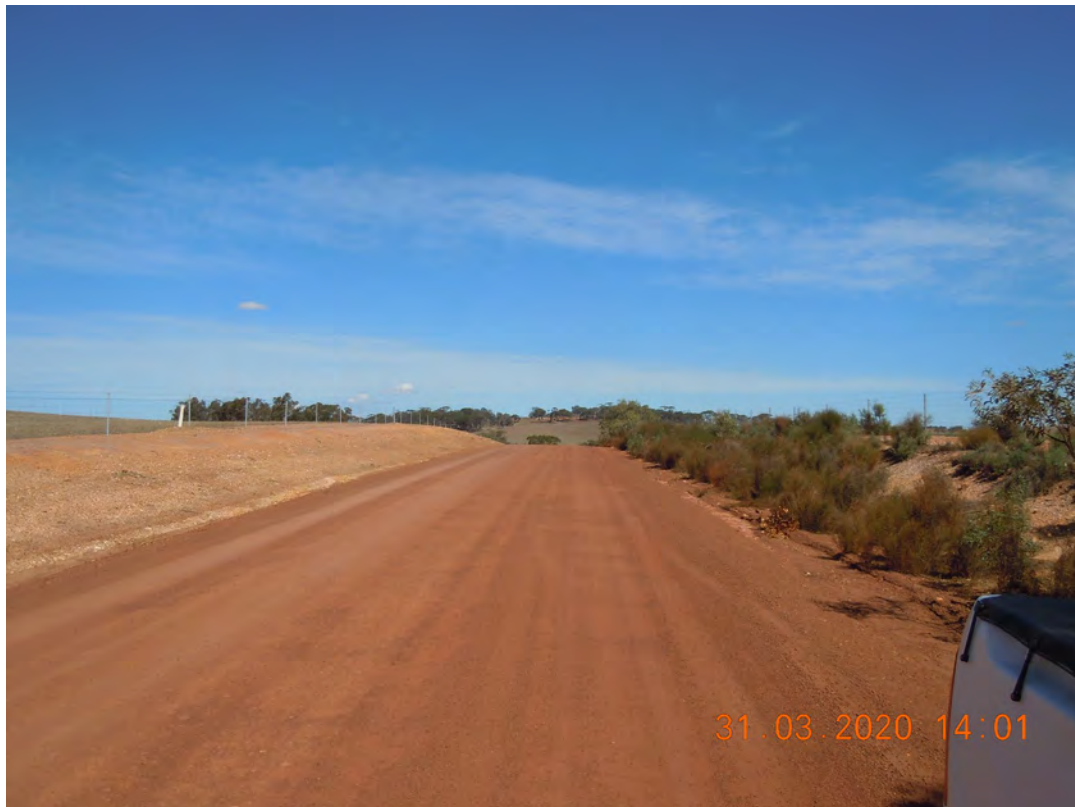
PHOTOGRAPH 16 2.04 SLK Cocking Road looking south
