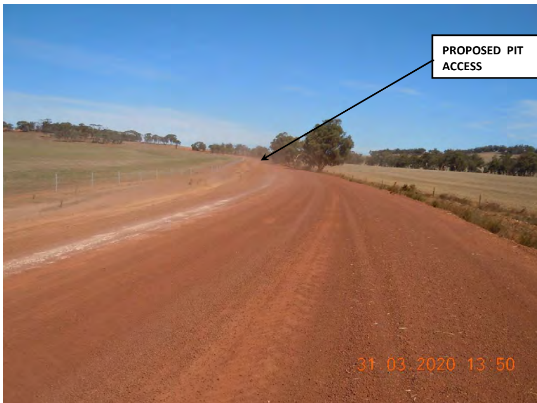
PHOTOGRAPH 2 SLK 2.56 Cocking Road Looking south
