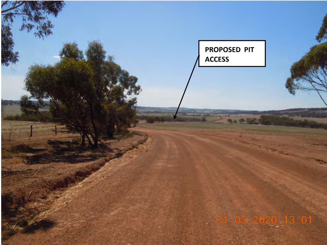
PHOTOGRAPH 1 - SLK 3.35 Cocking Road Looking north along Cocking Road south of proposed pit access
