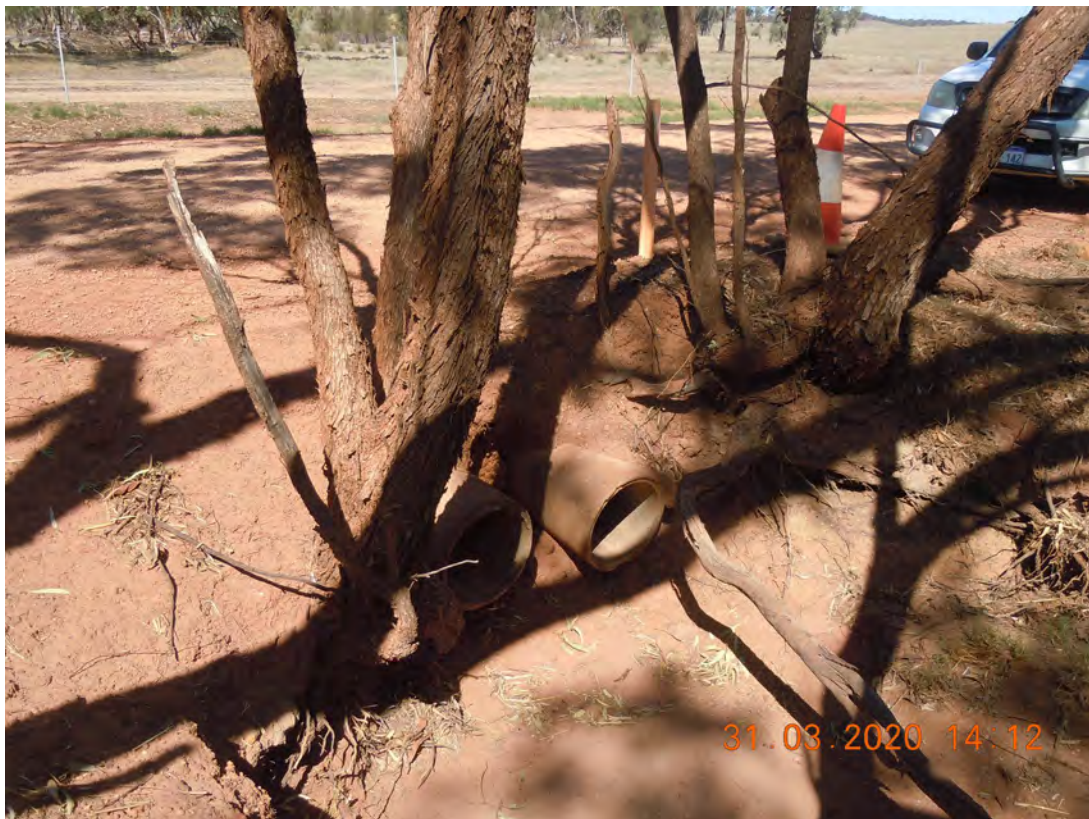
PHOTOGRAPH 22 - 1.22 SLK Cocking Road culvert LHS – mixed pipe sizes
