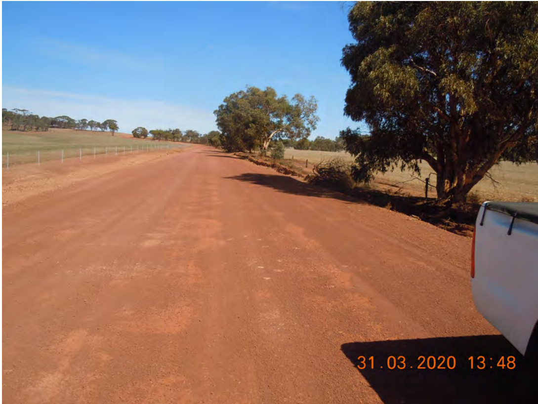
PHOTOGRAPH 9 2.66 SLK Cocking Road looking south
