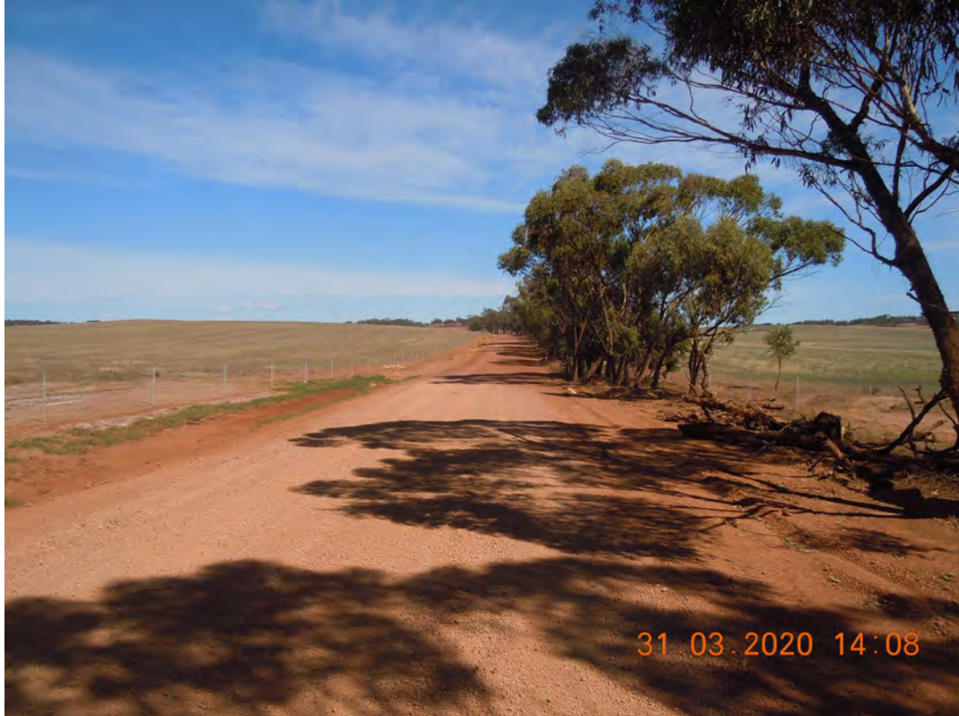
PHOTOGRAPH 20 - 1.22 SLK Cocking Road looking south from culvert
