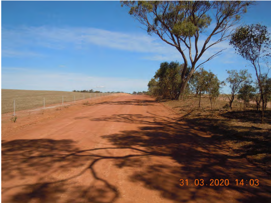
PHOTOGRAPH 17 - 1.92 SLK Cocking Road looking south
