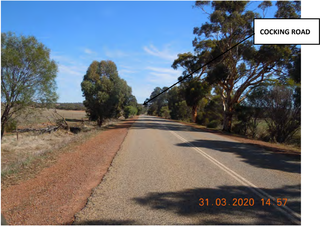
PHOTOGRAPH 33 - 6.62 SLK Mogumber Yarawindah Road looking west towards Cocking Road Intersection
