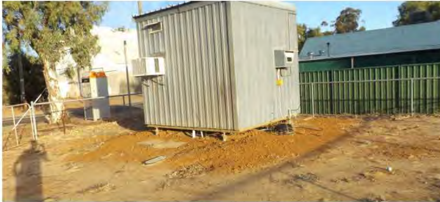
Photograph 1 – View of existing telecommunications exchange looking east across Denton Street.
