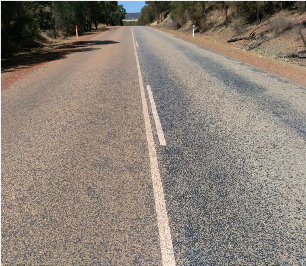
PHOTOGRAPH 13 7.51 SLK Looking West
