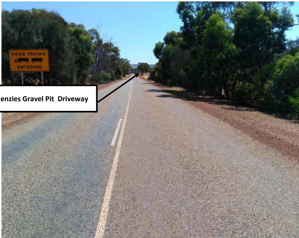
PHOTOGRAPH 12 7.51 SLK Looking East - Can see driveway at this point
