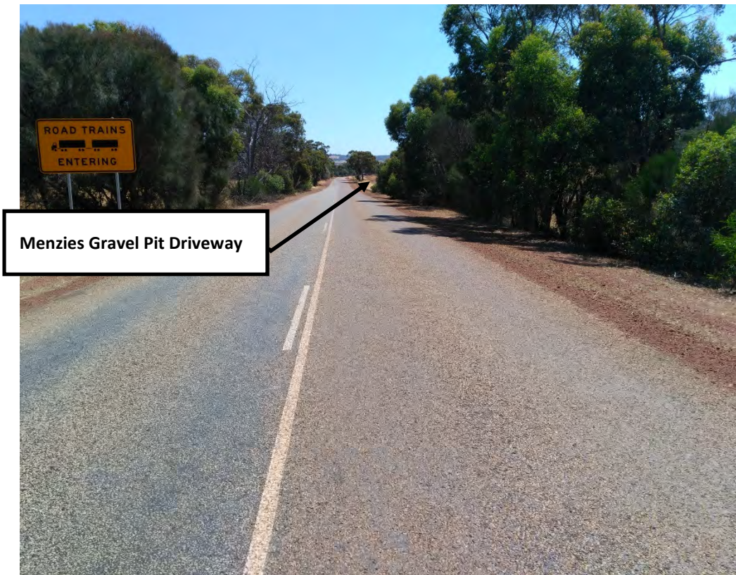
PHOTOGRAPH 3 7.51 SLK Looking East – Typical view of along the Mogumber Yarrowindah Rd
