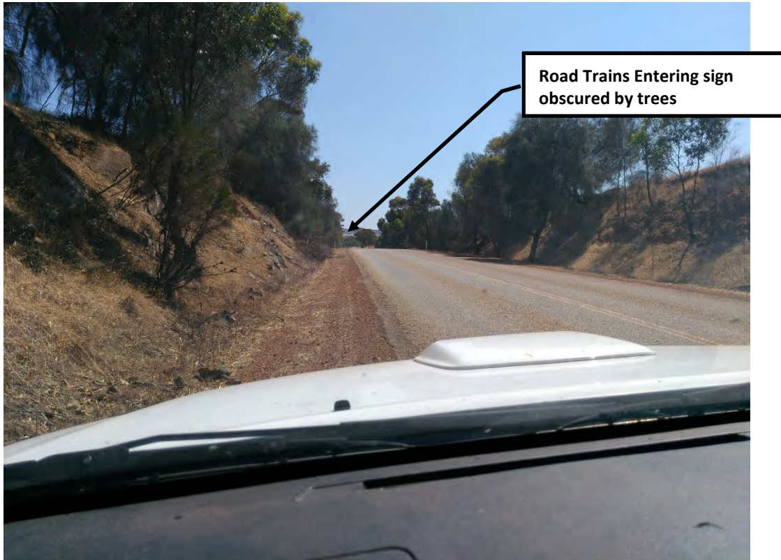
PHOTOGRAPH 10 "ROAD TRAINS ENTERING" sign on western approach along Mogumber Yarawindah Road obscured by trees
